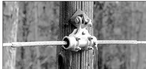
FIBERLIGN Cushion Clamp installed
